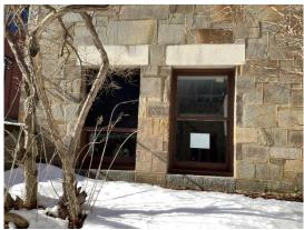
BE-26 The window to the right does not have an exterior storm, but one could be added. The window to the right serves as a vent.
