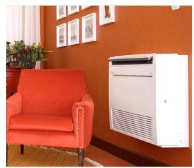
H-9 – Heat pumps offer different types of delivery equipment, such as this floormounted unit can be installed to be less obtrusive than the typical "mini-split" wall-hung units.
