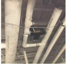
H-13 -- Pipes for Parish House (serves RE Wing, Metcalf and some uncontrolled areas) and Cloister (Offices) with controller for the Office zone.
