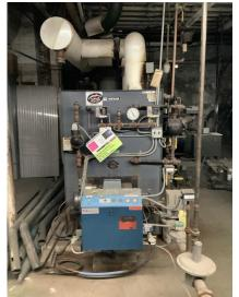
H1 — WUS has a large steam boiler that serves the entire building. Even if only 1 zone calls for heat the boiler must fire up so in a building with variable use patterns by zone, this is inefficient.
