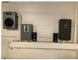
Photo E-7 – These lighting dimmers used to operate the Sanctuary lighting but were not replaced when lights were upgraded to LED, and are unlikely to be compatible.
