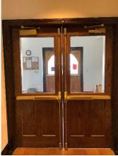
BE-13 – The RE wing has a vestibule that buffers heat loss between Metcalf Hall and the exterior
