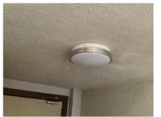
Photo E-5 – And LED surface-mount fixture in a hallway of the RE Wing.
