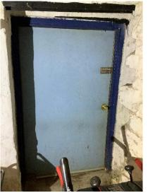
BE4 — Exterior door in the "snowblower room" needs weather stripping and 2inch poly-iso rigid insulation applied. Water pipes in this room need a heat tape and these improvements may eliminate it.
