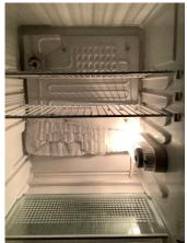
Photo E-11 – The small beverage fridge in the Symmes kitchenette was empty but set at such a low temperature that ice formed on the coils. Adjust to a warmer setting. Or turn it off until in-person events resume.
