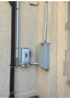
Photo E19 — The disconnect switch for the solar panels is located in the corner where the Metcalf Hall connects to the Office section
