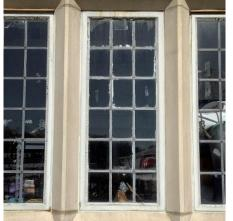
BE-18 -- This window in Metcalf Hall is the dominant window type: casement, single pane, leaded glass. Inefficient due to air infiltration and low R value.
