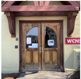
BE- 12 – The main door to the RE Wing has old weatherstripping that needs to be replaced, especially the gap between the two doors.
