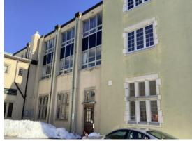
BE 17-- Exterior of the RE Wing. Large single pane windows with aluminum frames have poor thermal performance. The wall is stucco over cinderblock with no insulation.
