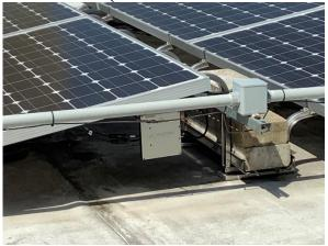
Photo E18 — The solar panels use Enphase micro inverters to convert the DC electricity generated by the panels into AC current usable by light, appliances, etc.
