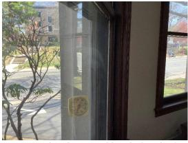
BE 16 – The view out this window in the Parlor shows wall construction: thick stone exterior, likely with little insulation between it and the interior wall.
