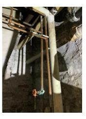
H-26 – The hot water pipes from the Ruud tank hot water heater are uninsulated, thus lose a lot of their heat on the long path to the Metcalf Kitchen and bathrooms. Insulating these pipes is a simple project with this insulation readily available at the hardware store or home center.
