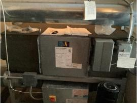
. H-23 – An energy recovers ventilator (ERV) serves the Meyer Chapel, located in the Mourning Room, providing dehumidification and fresh air during times of high activity. It brings in outside air while transferring heat from the exhaust air.
