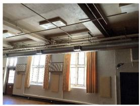
H-25 – The new duct work in Metcalf Hall (above the windows) connects to an ERV for dehumidification and fresh air in this space.
