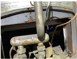
.H-5 -- Pilot light for the hot water heater burns gas 24x7x365.
