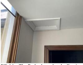
BE-14 – The Parlor has a hatch allowing access to space above the dropped ceiling which should enable adding insulation
