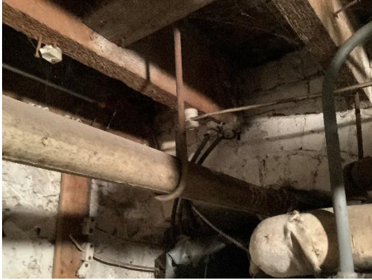
E1- Knob-and-tube wiring Example 1
