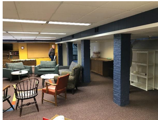
E5- Jr High classroom- fluorescent light fixtures
