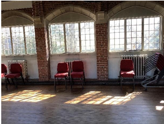
BE7 - Rectangular windows in arched openings could be upgraded to double or triple pane.
