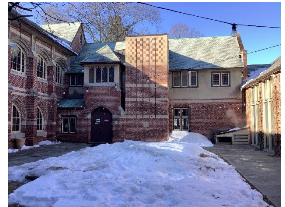
Parish office entrance
