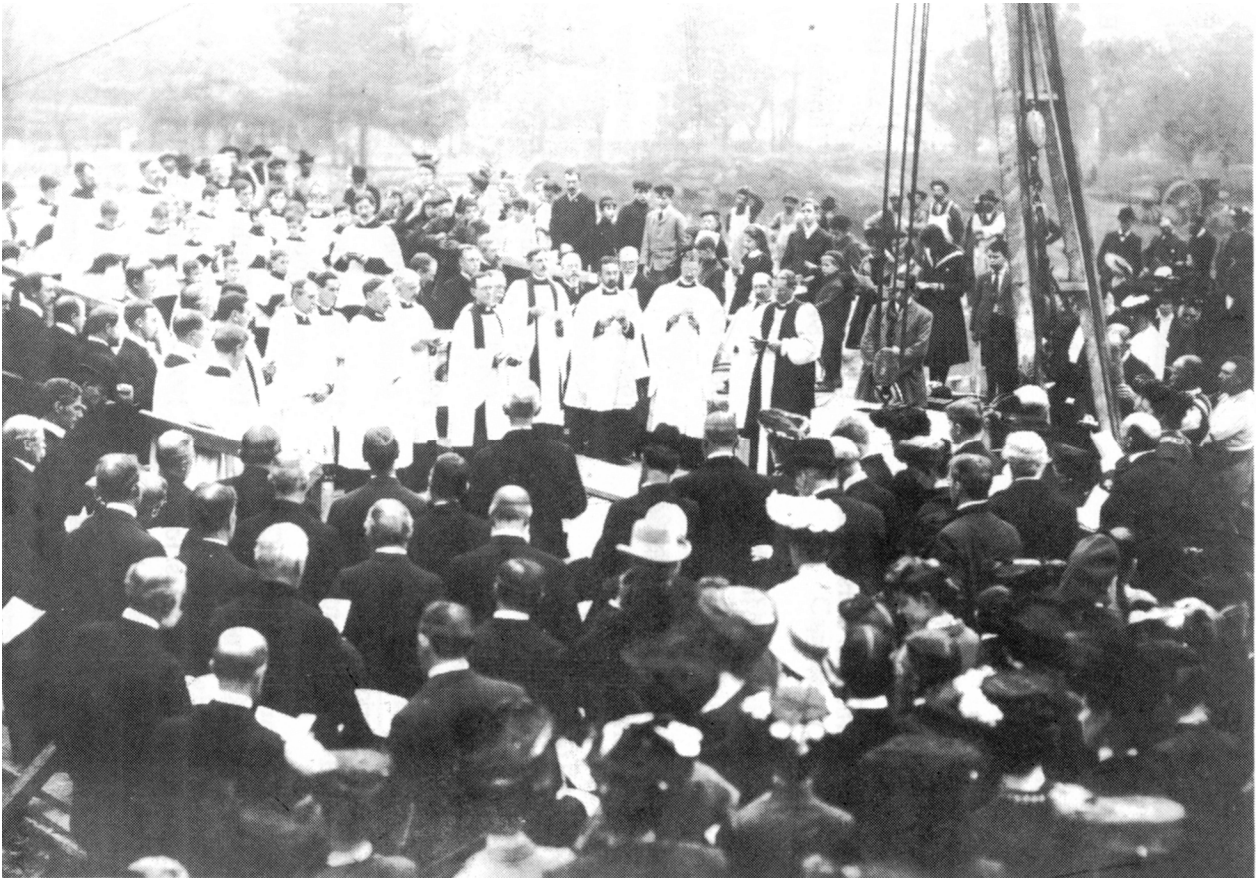
Laying the Cornerstone: October 20, 1904
